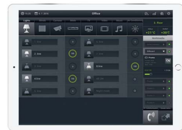
Control via tablet
