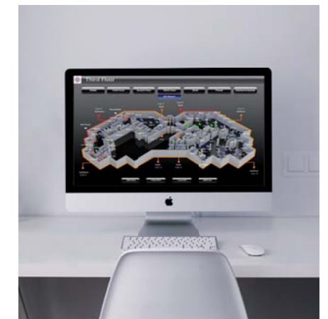
Building management system
